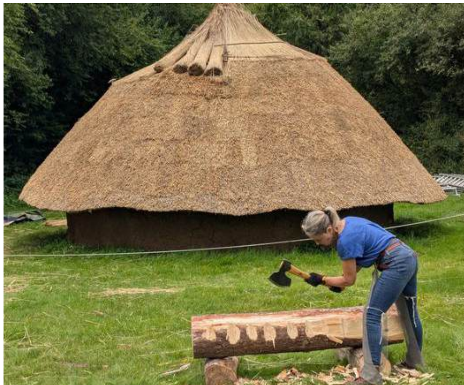
The Roundhouse Project underway at West Stow Anglo-Saxon Village.
