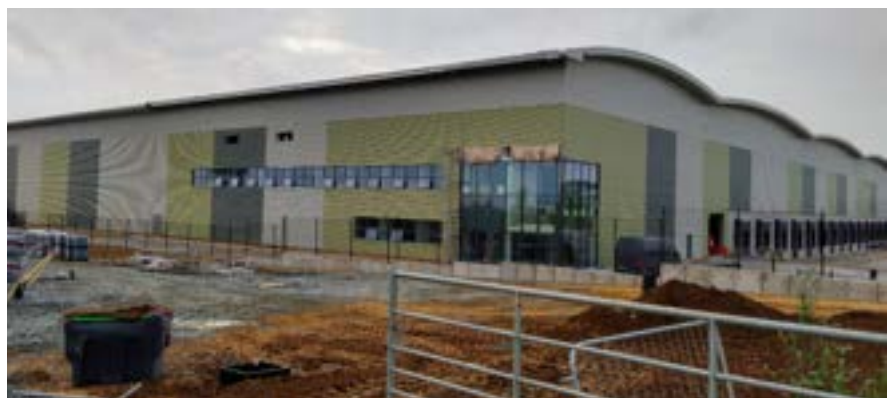
The giant warehouse under construction at the Suffolk Business Park.
